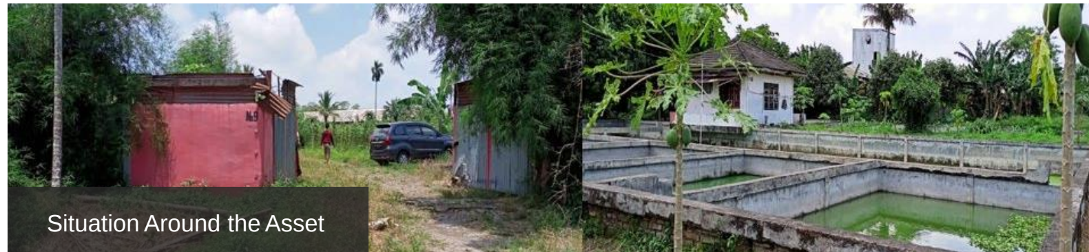
Situation Around the Asset
